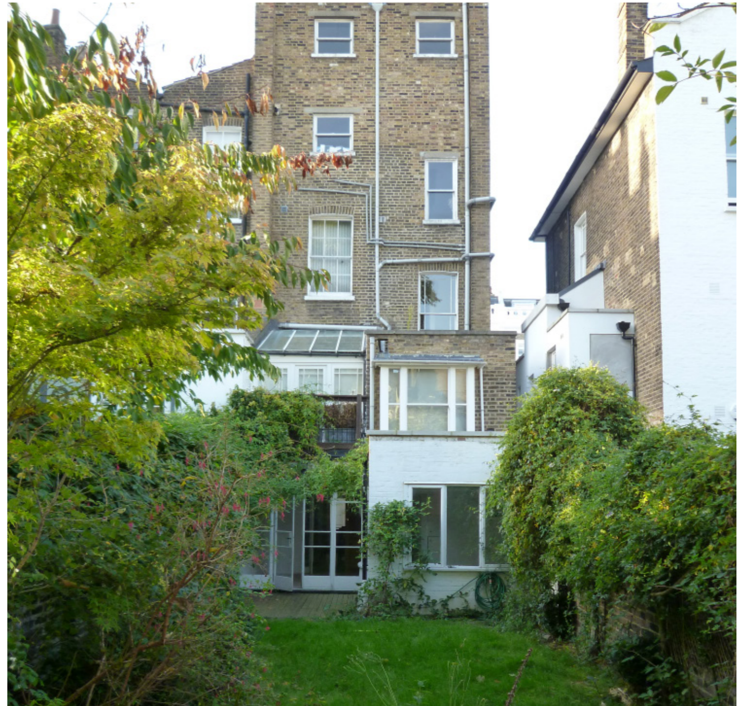
Photograph of the back facade of 5 Fitzroy Rd.
