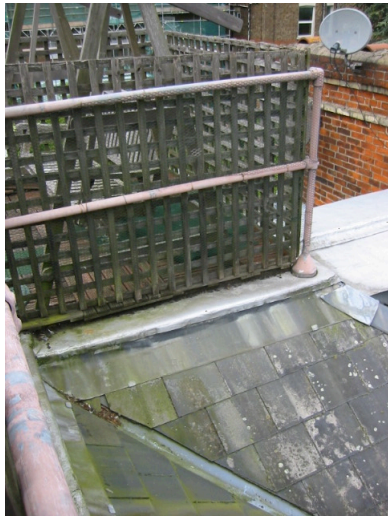
Existing railing - Key Clamp handrail, painted pink, with guarding panels of timber garden trellis
