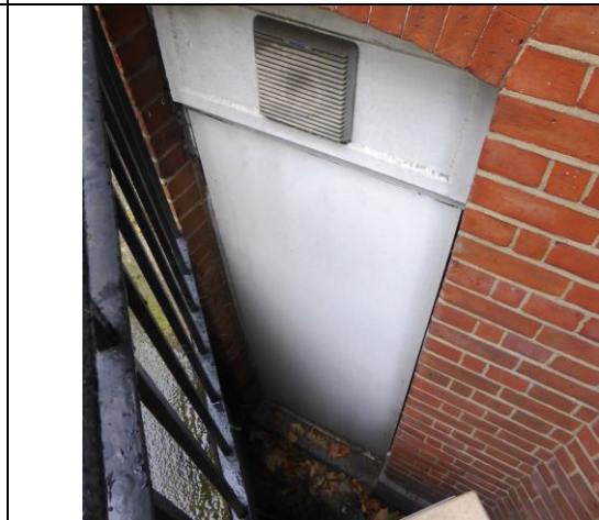
Fig 6 Existing Basement Photocopy Room boarded over door to Lightwell
