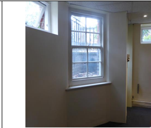
Fig 2 Existing Basement Photocopy Room & Sash window to Lightwell
