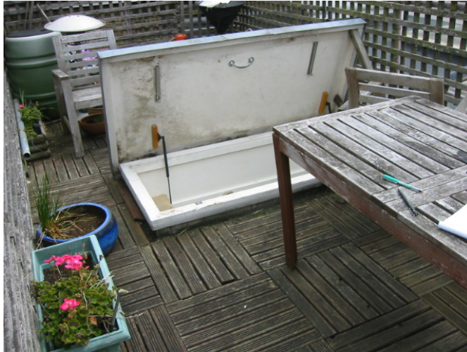
Current, hinged, roof access
