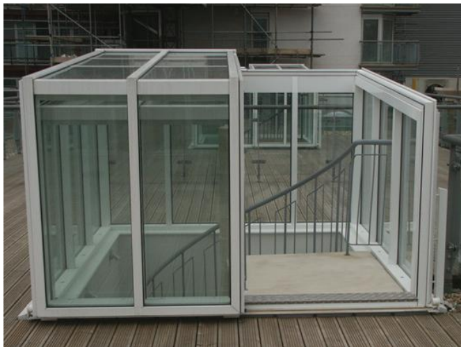
Proposed sliding lantern roof access
