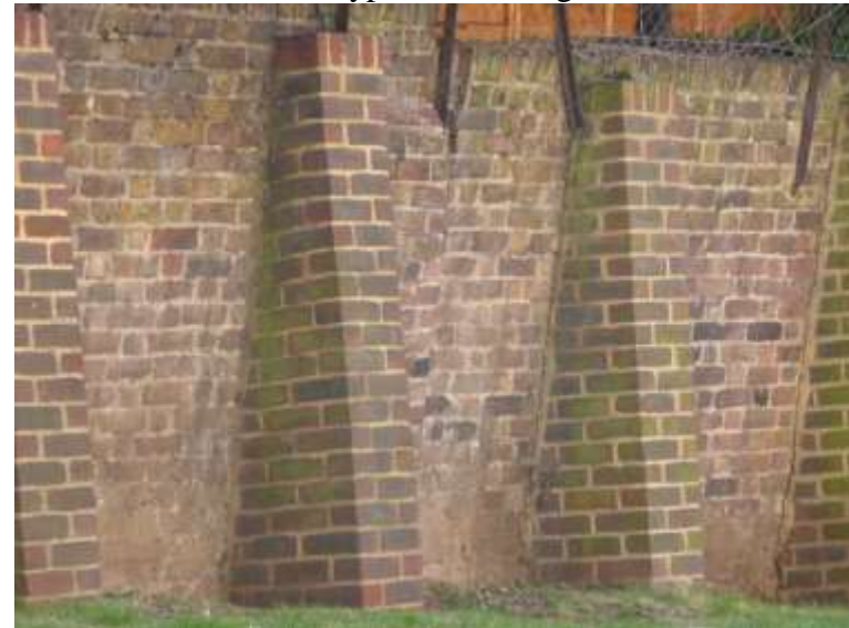
8. Illustration of Loss of Verticality
