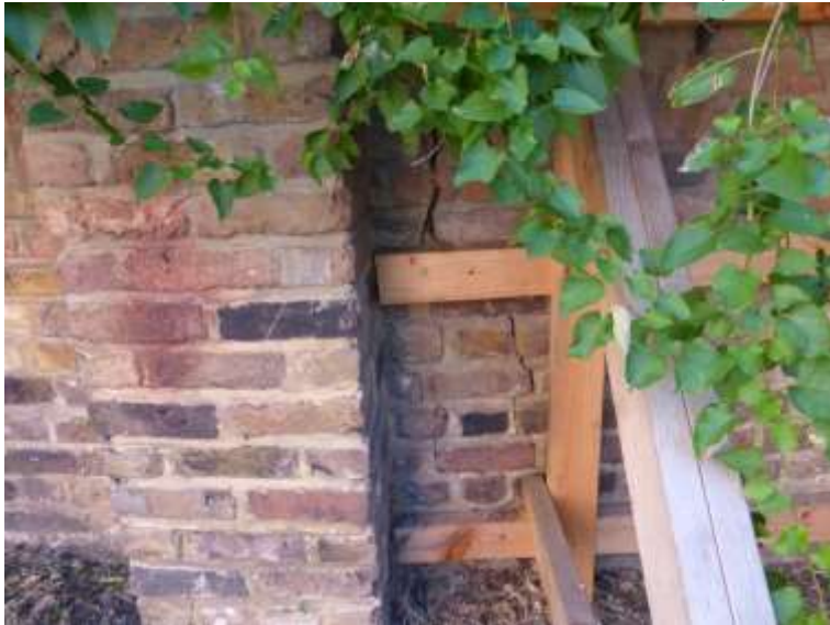
5. Typical Crack
