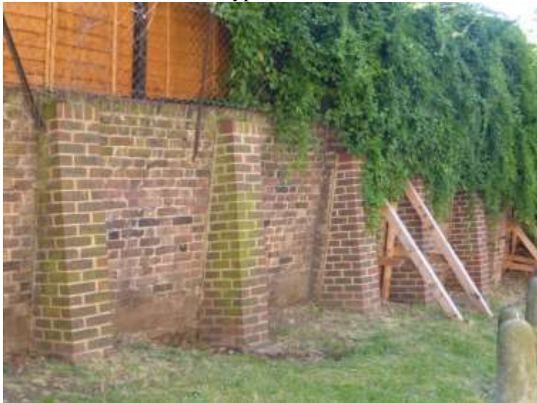
7. Illustration of Loss of Verticality
