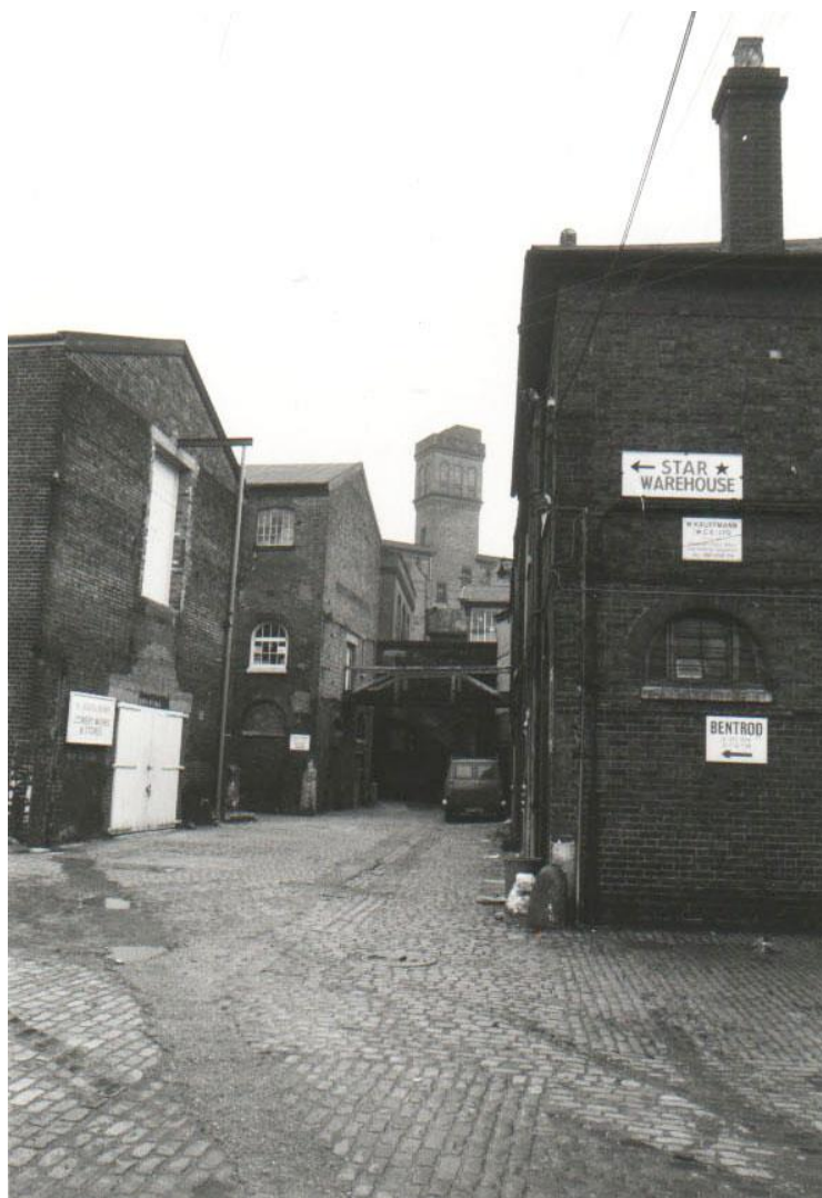
Figure 7 1975 photograph showing the bridge.
