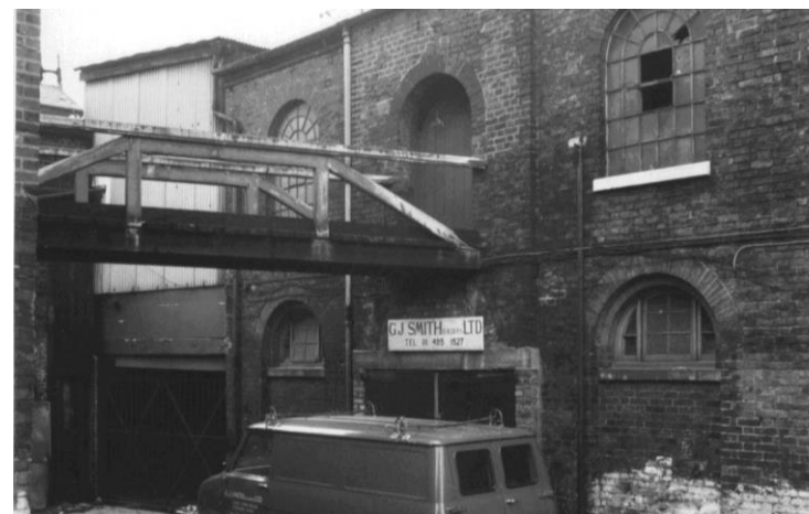
Figure 1 The Tack Room showing the bridge in 1975 before its removal.
