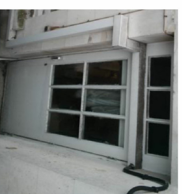
Existing Panel above door to be replaced with louvre.
