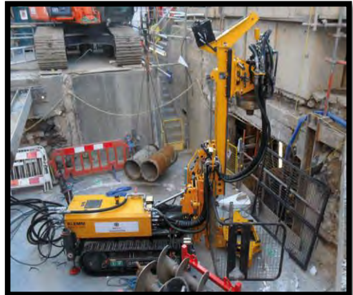
Non percussion/vibrating rig
