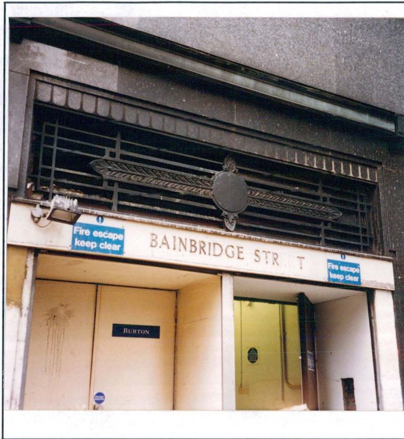
REAR EXIT- BAINBRIDGE STREET (NOTE OVERHEAD GRILL)
