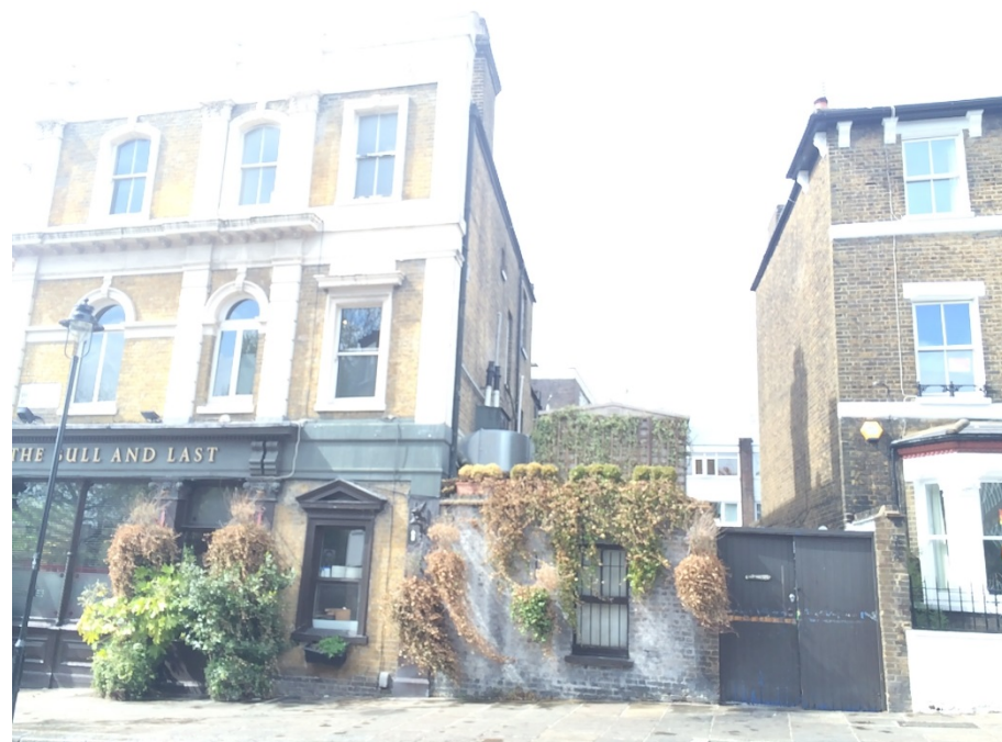
Photograph 5 –Side Passage Elevation
