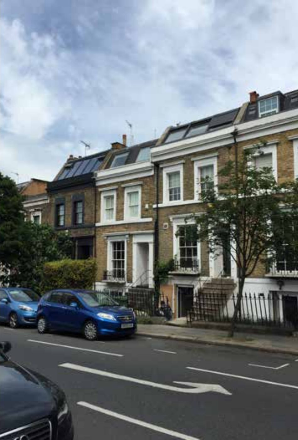
Precedent - Glazed set back on sloped roofs on Victorian terraces (in Kentish Town)
