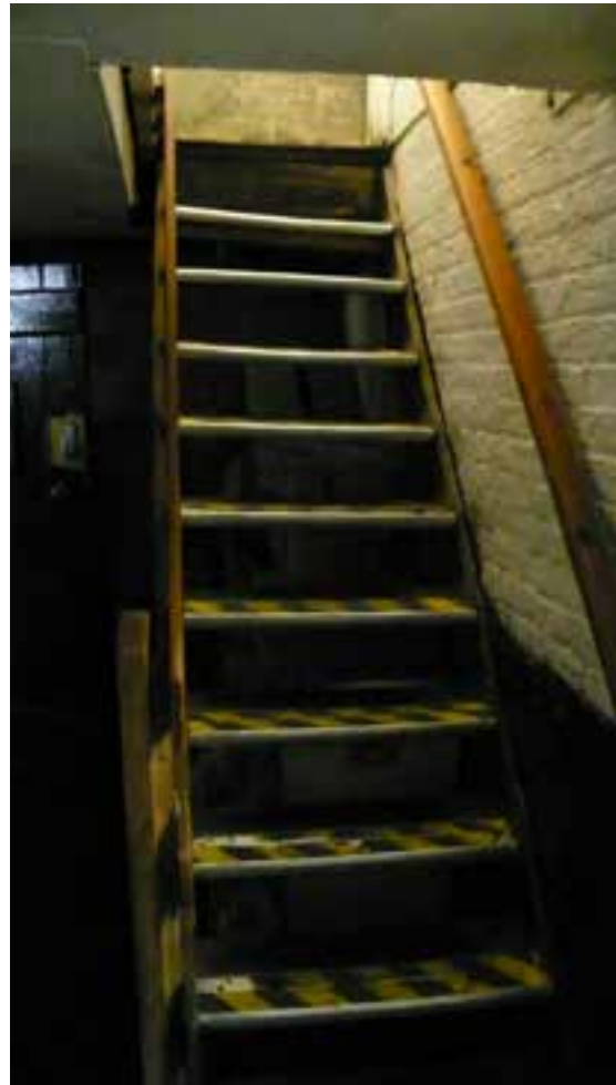
Existing basement stair
