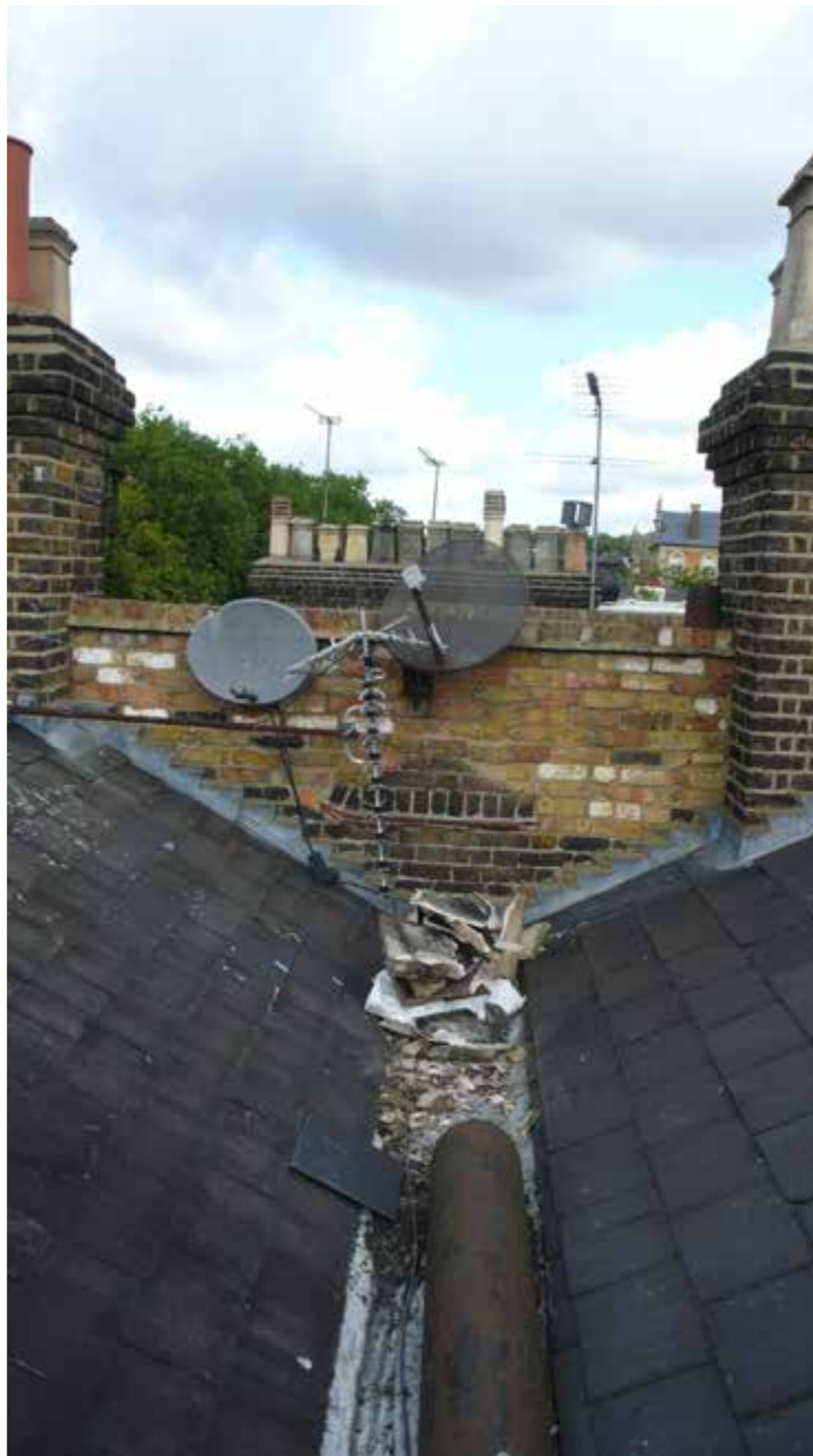
View of the existing valley roof
