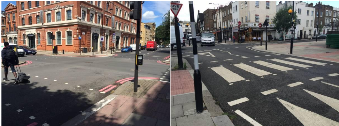
Figure 3.4 Camden St / Plender St (left) and Plender St / Bayham St (right) junctions
