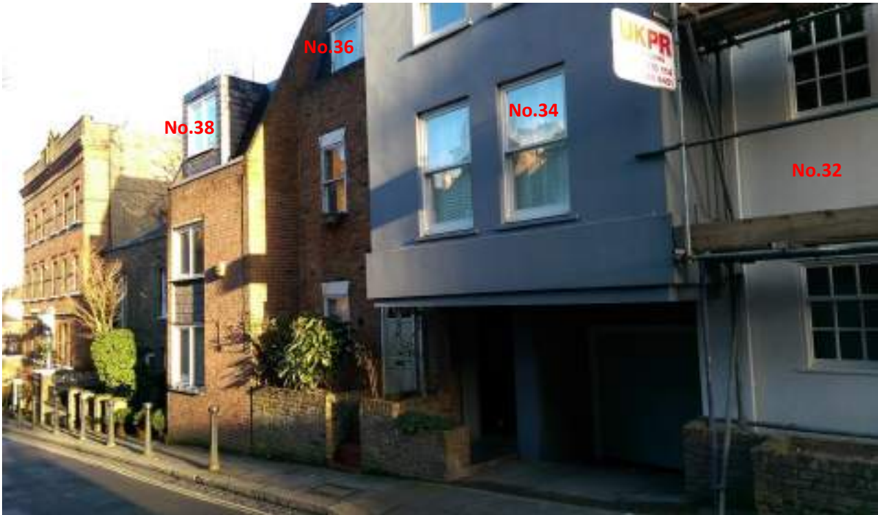
Photo 1: Front elevation (street scene) looking east. No.36 Flask Walk is a 3 storey terraced house with a mansard roof. There is a communal covered parking area which is shared by No's 30-36, and can be accessed via the garage door and ramp located beneath the adjoining No.34.
