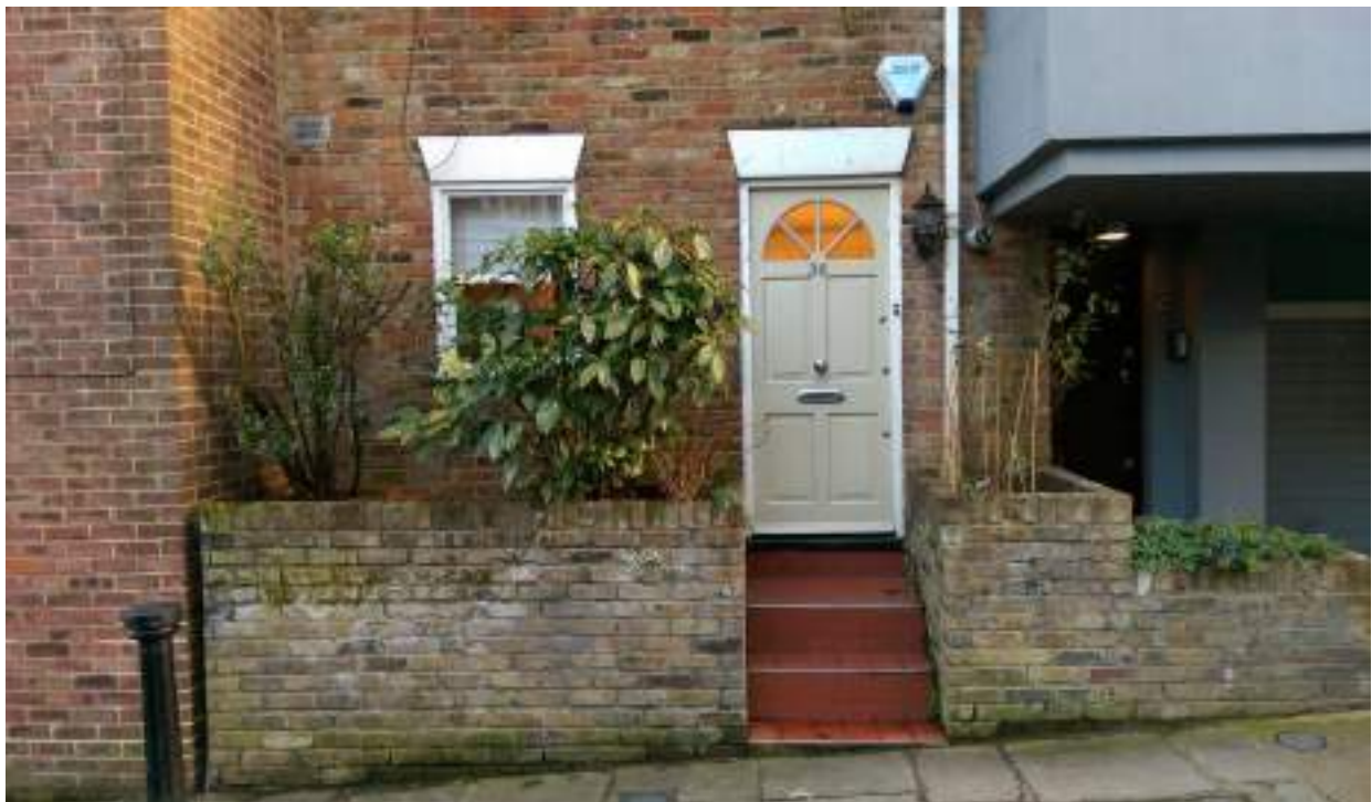
Photo 4: At the front of the property there are two raised planting areas, and a short flight of steps which lead up from the footway.
