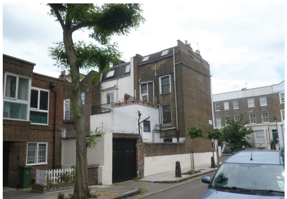
Side and rear elevation of 28 Grafton Terrace
