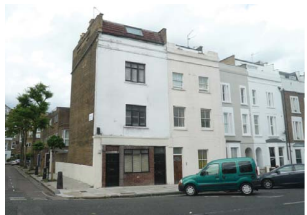
Front elevation of 28 Grafton Terrace
