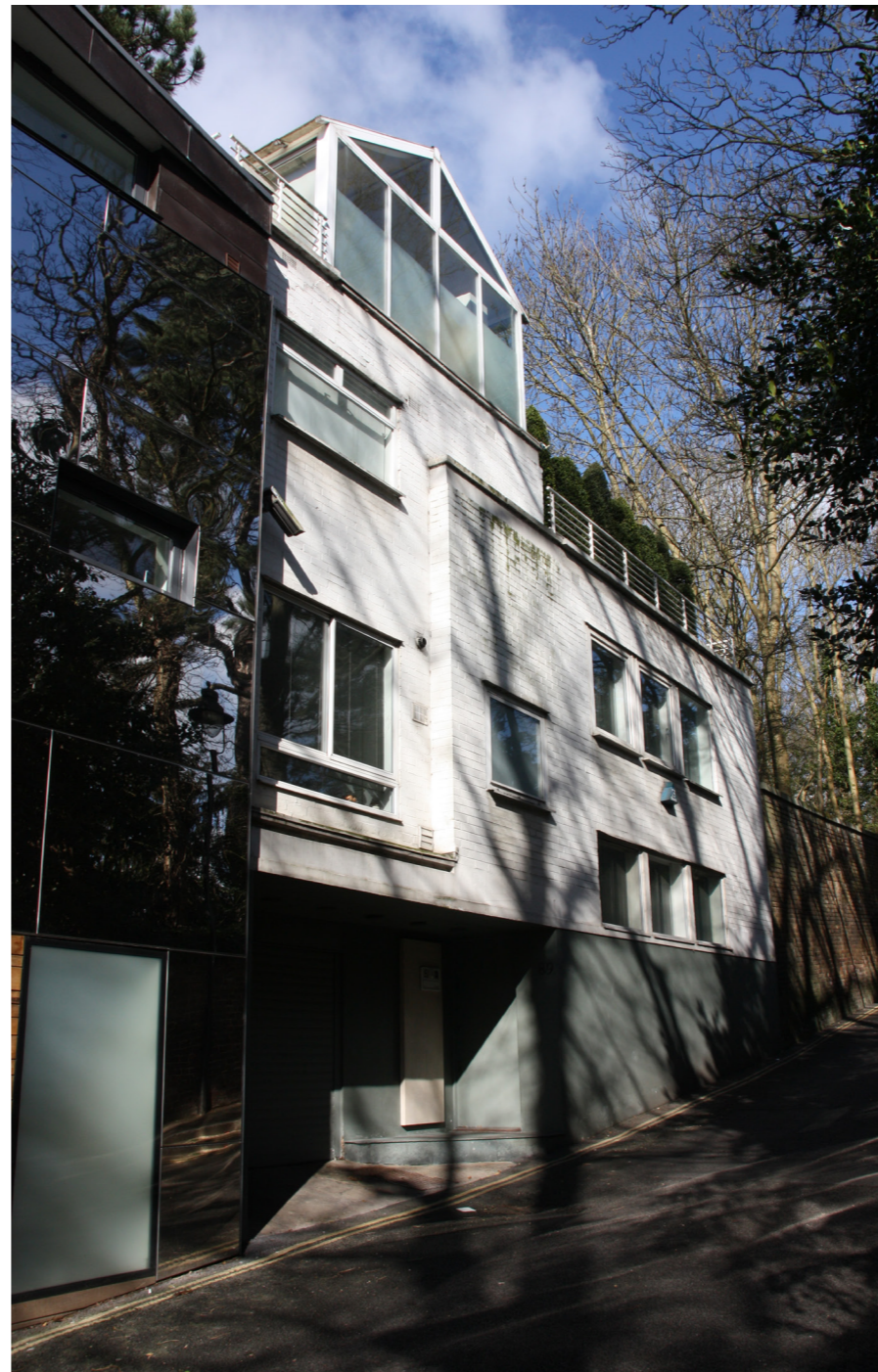
No. 89 with the reflective cladding to no.87 in the foreground
