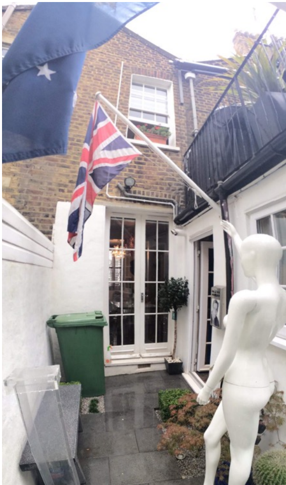
Rear elevation of 1 Kelly Street.
