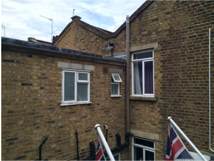
Back addition of No.3 Kentish Town Road- from back addition roof.
