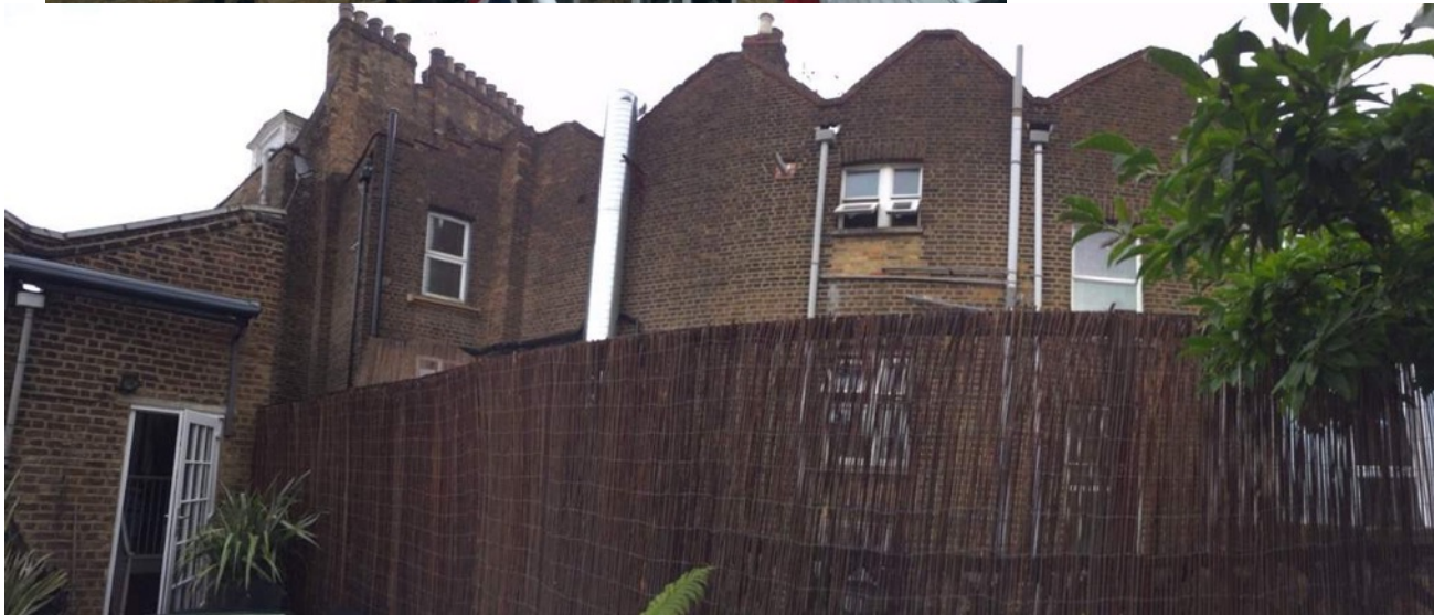
Rear elevations of properties on Kentish Town Road from back addition roof.
