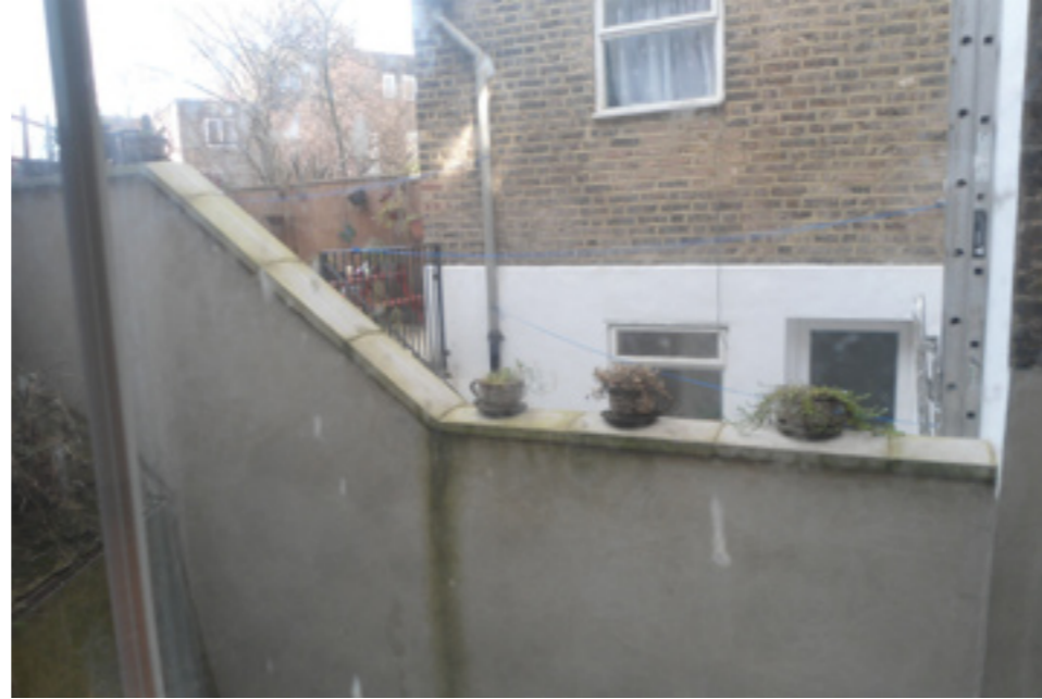
North site boundary in number 121
