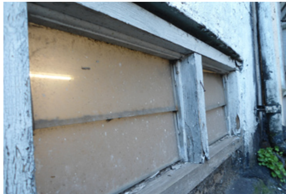
Ground floor kitchen window in number 119
