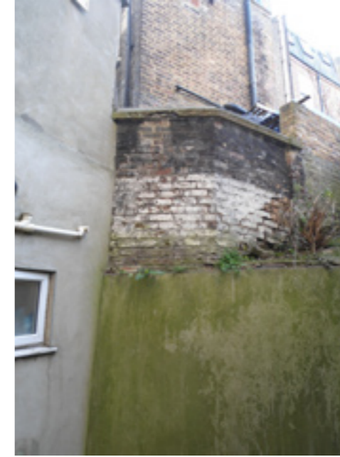
Basement patio in number 121
