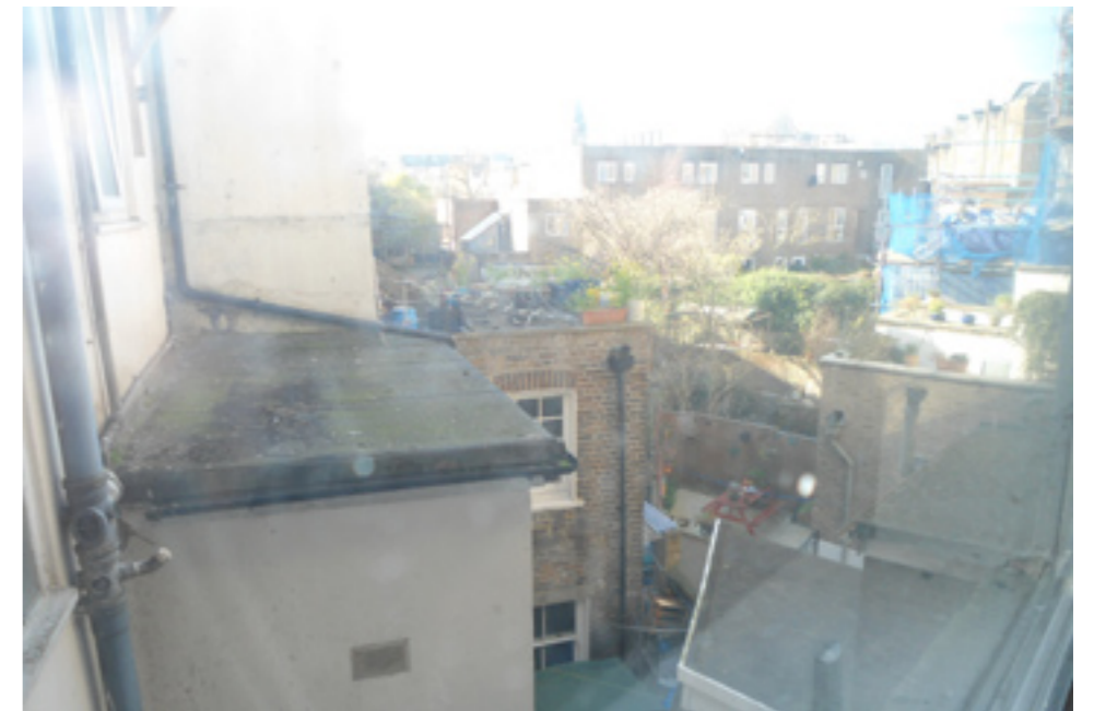
View of the block courtyard from the corner of 119
