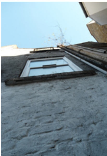
View of the rear facade of number 119
