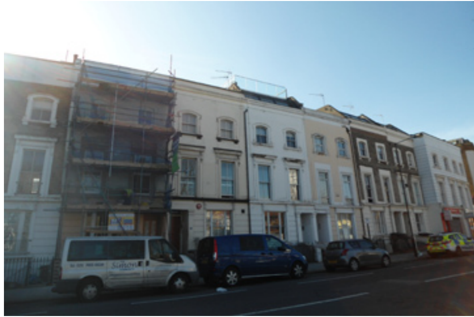
Malden Road 127 with scaffolding
