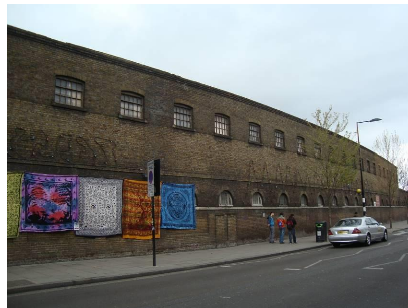
Figure 3 The 'Camden Wall', Chalk Farm Road.
