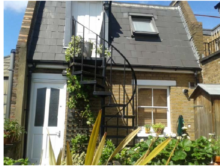
8. Rear view of No.166 showing existing rear fenestration
