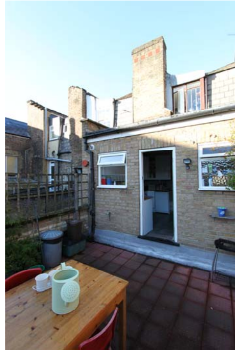
5. Rear view of No. 164a and No.162 on LHS
