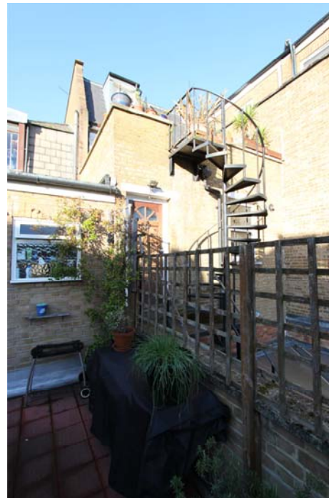
6. Rear view of No. 164a and No.166 on RHS
