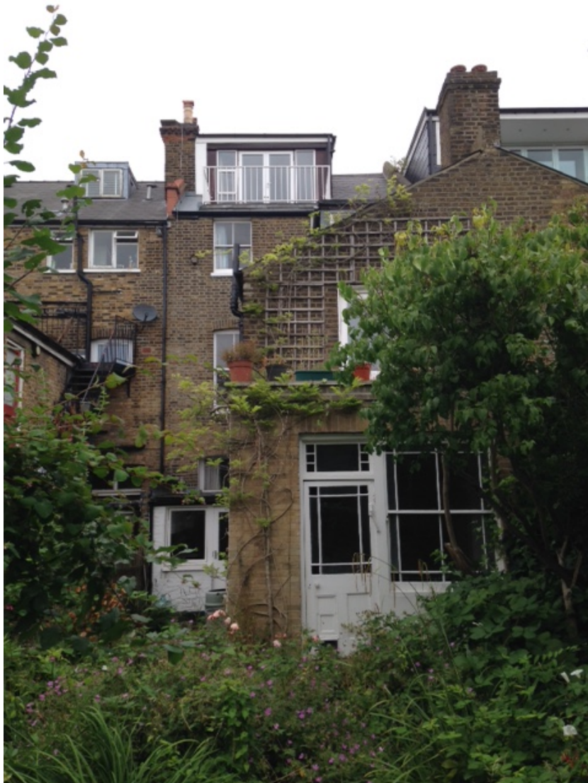
Fig.2. View of existing rear elevation
