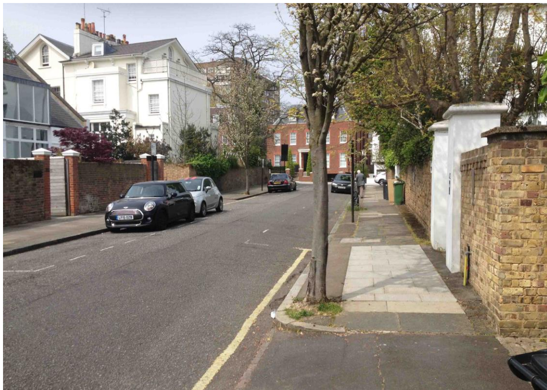
Photo 4: The Woronzow Road carriageway immediately to the west of No.34 falls gently towards the south. Note the fall of the footway towards the carriageway, away from the property.
