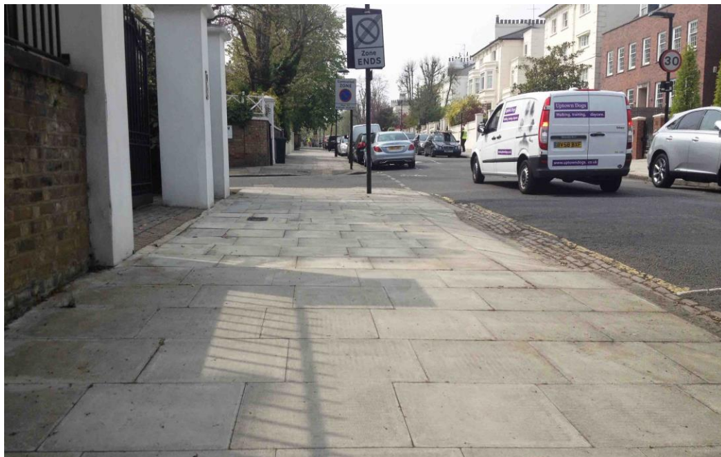
Photo 2: The footway in front of No.34 falls gently towards the Queens Grove carriageway, away from the property.
