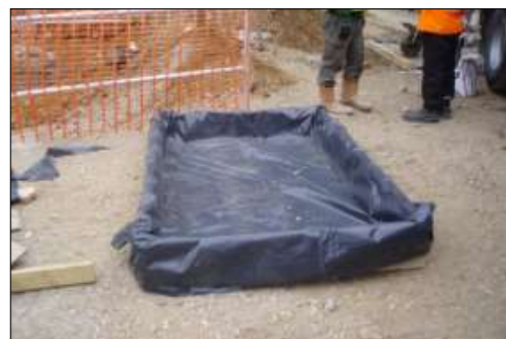
Photo 47: Soil bunding or a supporting framework covered in heavy-duty plastic sheeting is essential where there is a risk of spillages contaminating RPAs. This specifically applies to cement mixing areas and vehicle washing facilities.
