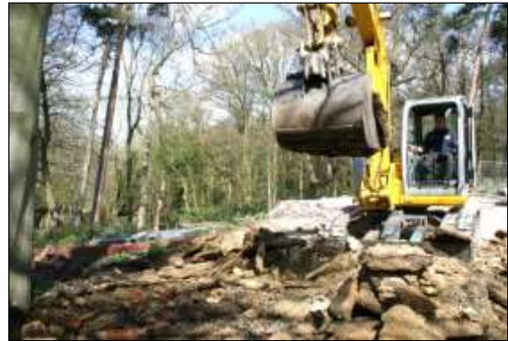
Photo 20: Machines with a long reach can be used to lift out heavy surfacing and structures as long as the machine sits outside the RPA and the exposed surface is protected before there is any further access.
