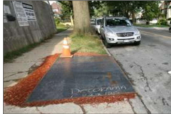
Photo 14: Steel plates can be an effective way of temporarily reinforcing weak surfacing over a construction access during the development activity.
