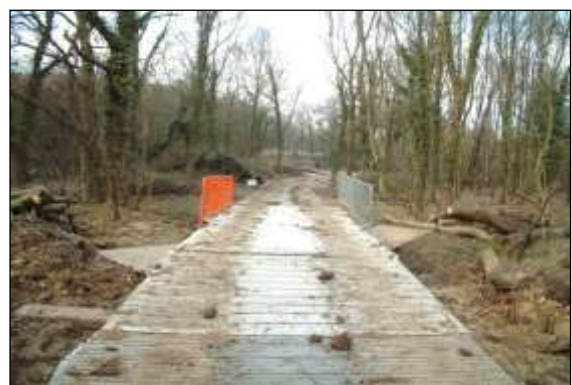
Photo 12: Custom designed sectional tracks can be joined to support very heavy traffic use through sensitive areas.
