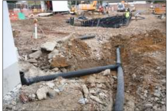
Photo 56: Drainage from adjacent buildings can be directed into Silva Cells, significantly buffering rainwater runoff from urbanised areas.
