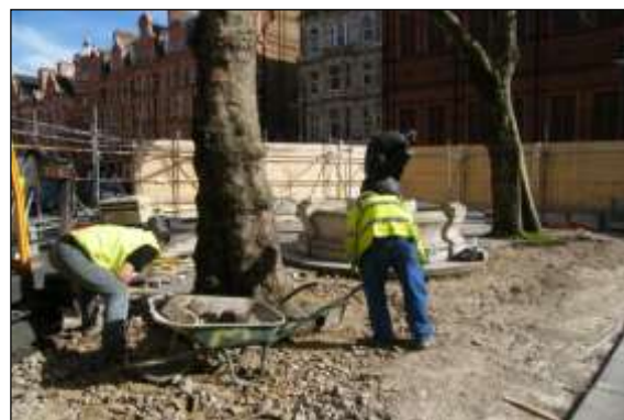
Photo 22: These trees had impermeable surfacing right up to their trunks, which had to be removed by hand before installing new structures.
