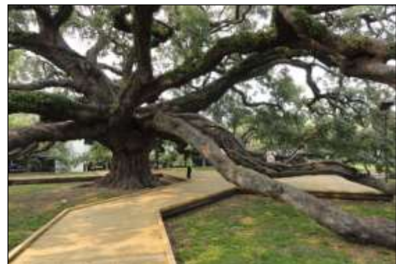
Photo 31: Board walks supported on posts or a light frame are another way of providing pedestrian access across sensitive RPAs.
