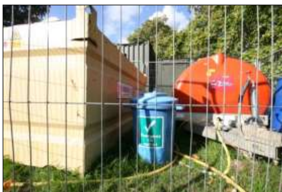
Photo 46: Where fuel or other chemicals are stored on site, it is now standard practice to have emergency spillage kits available to restrict the environmental impact of accidents.
