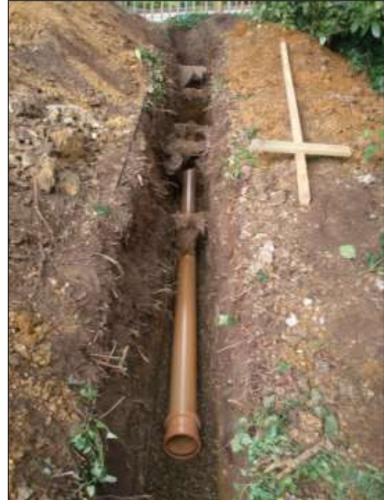
Photo 45: Continuous trenches dug by hand so that important roots can be retained (with the service ducting threaded beneath) is an effective means of minimising damage (note the ground protection boards with soil piled on top on the left).
