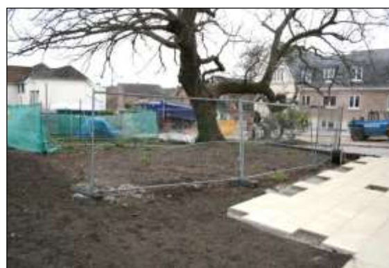
Photo 49: This tree had tarmac parking within its RPA that was removed and replaced with an organic mulch near the trunk and limited no-dig surfacing on the outer edges of its RPA.
