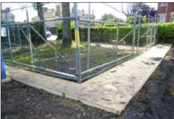
Photo 9: Plywood fixed to a wood frame is another effective method of protecting soil from pedestrian compaction.
