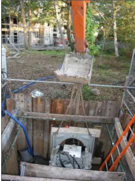
Photo 44: If possible, thrust boring is the preferred option for installing service routes through the RPAs of important trees, but there has to be space at the start and finish to dig substantial working pits.
