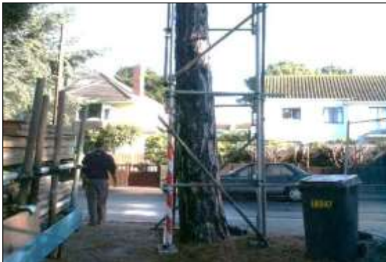
Photo 5: A scaffold braced framework surrounding the trunk reduces the risk of accidental impact.
