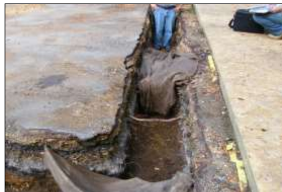
Photo 18: Exposed roots must be protected from light, drying out and extremes of temperature by covering with hessian sacking and boards until they can be covered back with soil.
