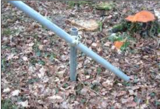
Photo 3: Close up of bracing detail, essential for increasing the stability of the vertical framework.
