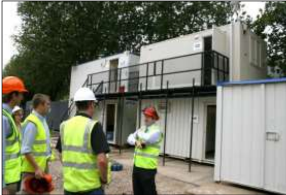
Photo 13: A combination of retaining existing surfacing and using temporary construction cabin accommodation can be a very effective means of preventing damage to sensitive areas.
