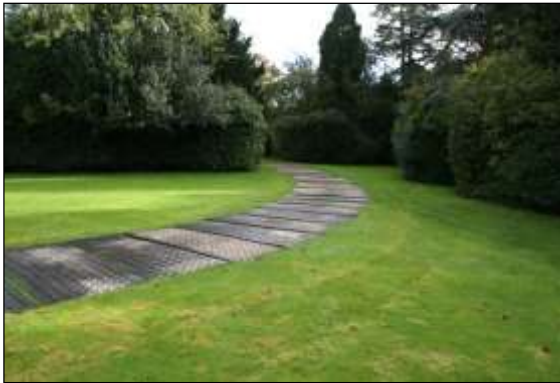
Photo 19: Ground protection must be used where repeated foot or vehicle traffic could cause compaction in sensitive RPAs. It can be as simple as plywood for pedestrians, but must be more robust for vehicles.
