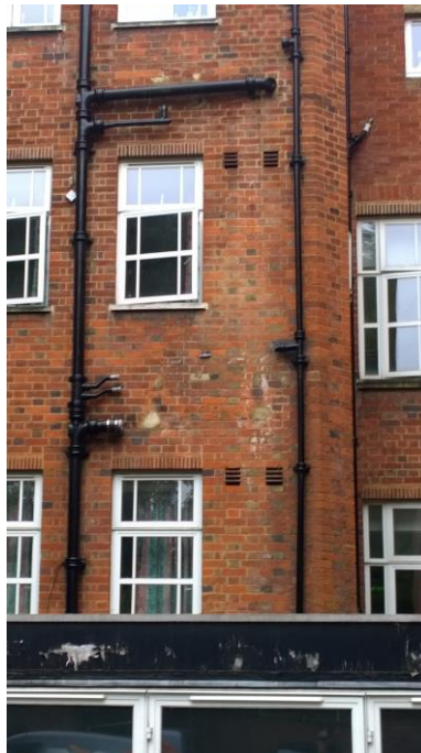
Photograph 9 Clay tile louvered vents on northern elevation of B1.
