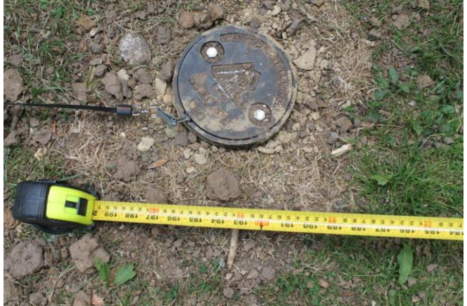
Photo 2. Monitoring point at 0.9m from the end of QMH dictated the max extent of the trenching. Smaller tape is to allow the roots to be plotted.
