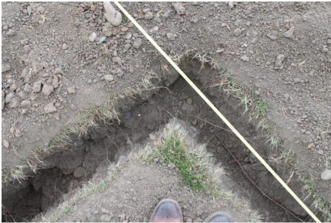
Photo 9. Trench 3 between 5.1m and 5.8m from the start of the trench.
