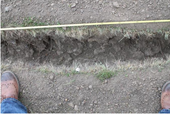
Photo 7. Trench 3 between 3.5m and 4.5m of the start from the trench.
