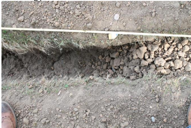
Photo 3. Trench 3 between 0m and 0.5m from the monitoring point.
