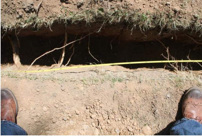
Photo 13. Between 10 and 11m from QMH is one 35mm root, one 11m root and 3xN° 5mm to 8mm roots.
