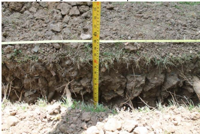
Photo 8. Ground was very hard clay. Even after terraventing to break up the soil the excavation had to cease at approx. 300mm -350mm depth
