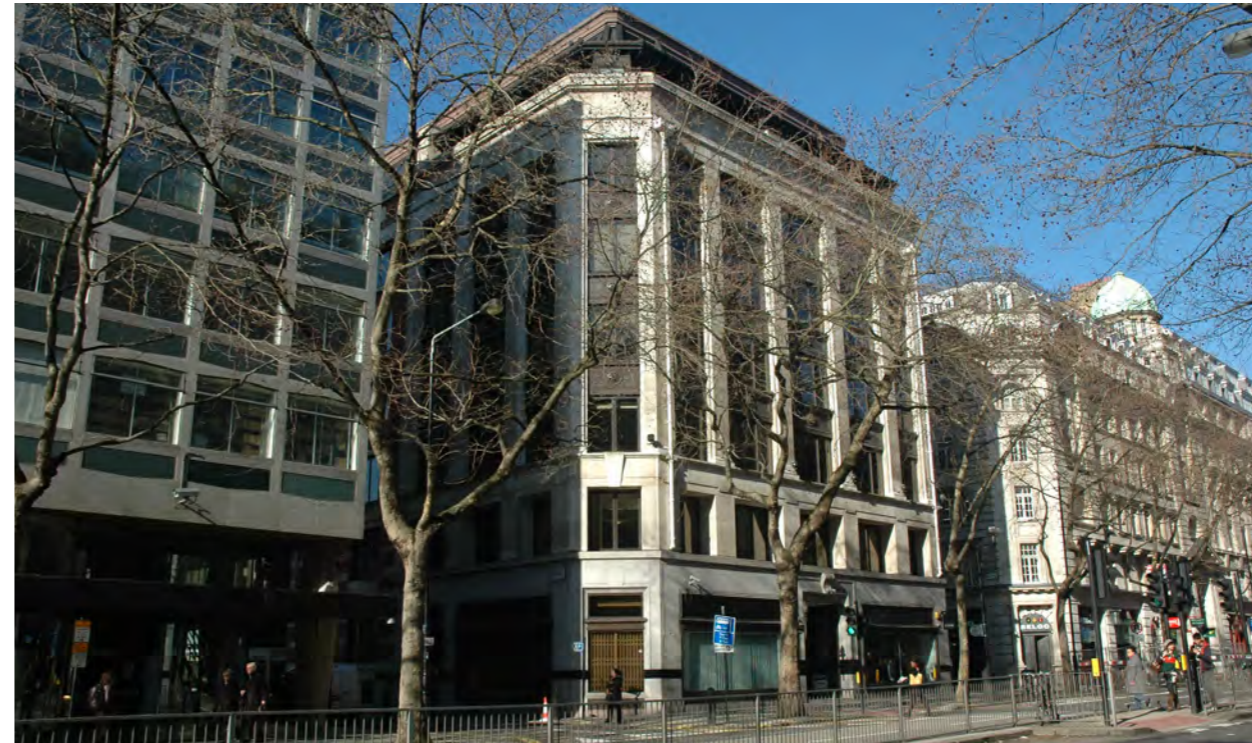
fig 1.1 External image of 65 Kingsway
