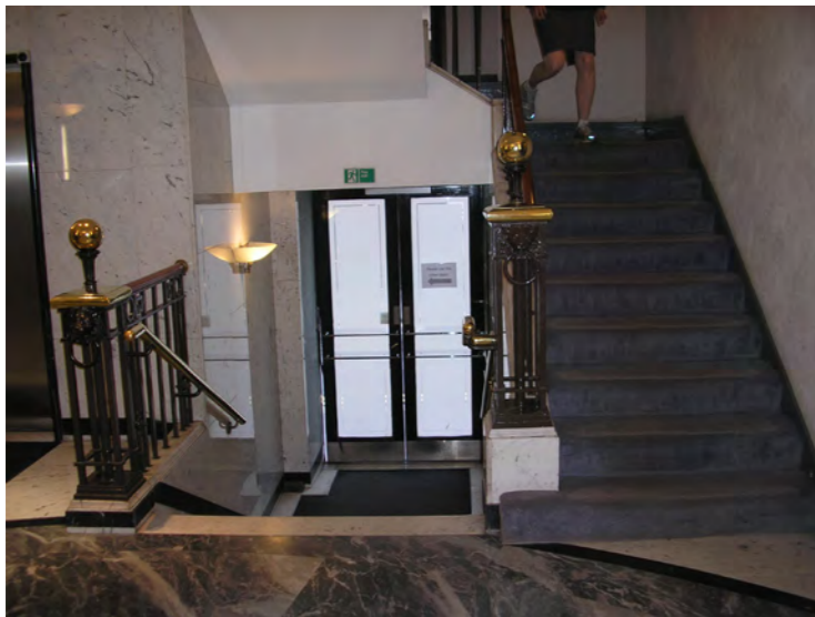
Existing stepped entrance from Wild Court
