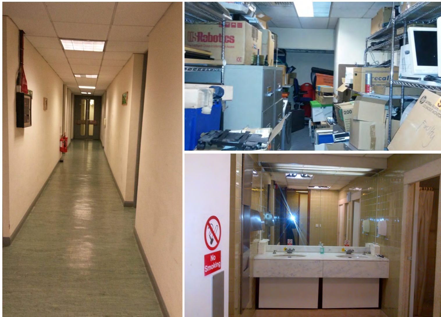
Typical existing basement areas and existing basement shower areas
