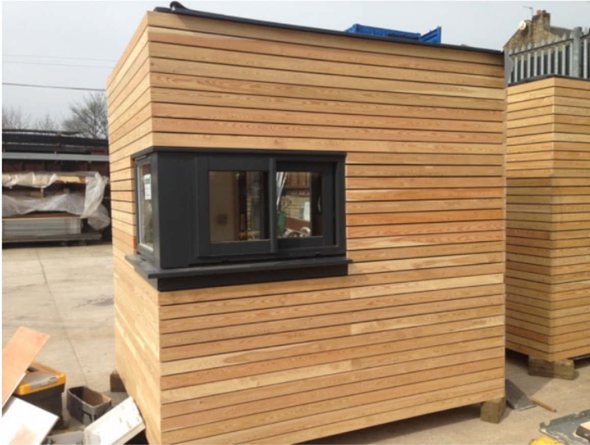
Example of pre-fabricated outbuilding
