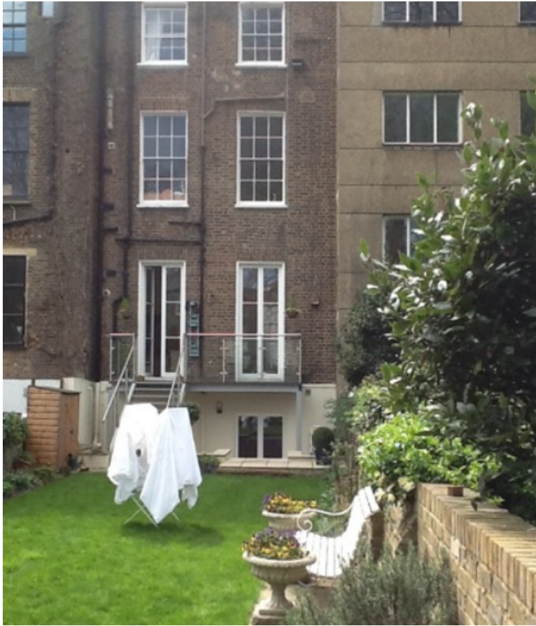
View back to the existing building.
