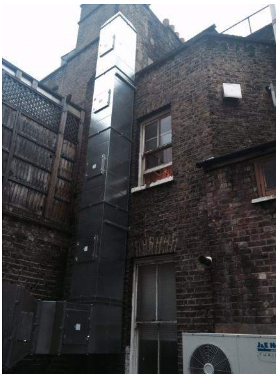
Figure 2.2 – Existing Flue Stack
