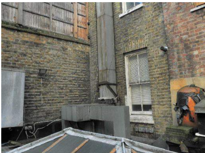
Figure 2.1 – Previous Flue Stack
