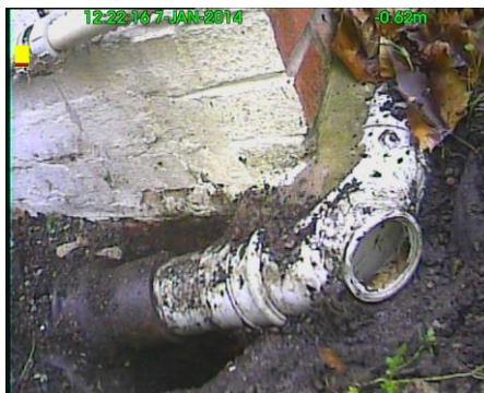
Pipework to WC is visible at ground level
