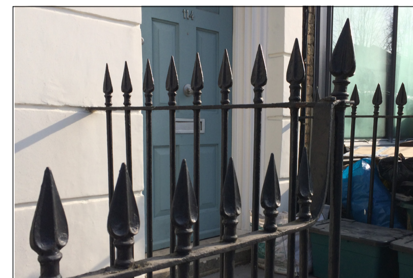
Images of adjacent railings
