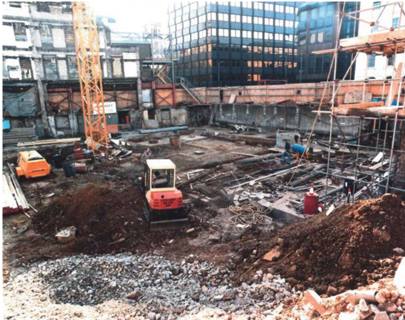
Archive image of Bloomsbury Plaza Under Construction (1980s)
