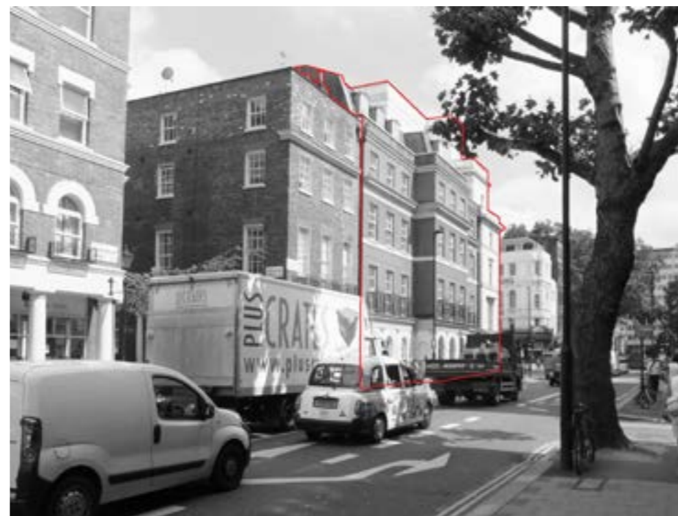
4. Looking South along Bloomsbury Street. Adjoining 10 Bloomsbury St
