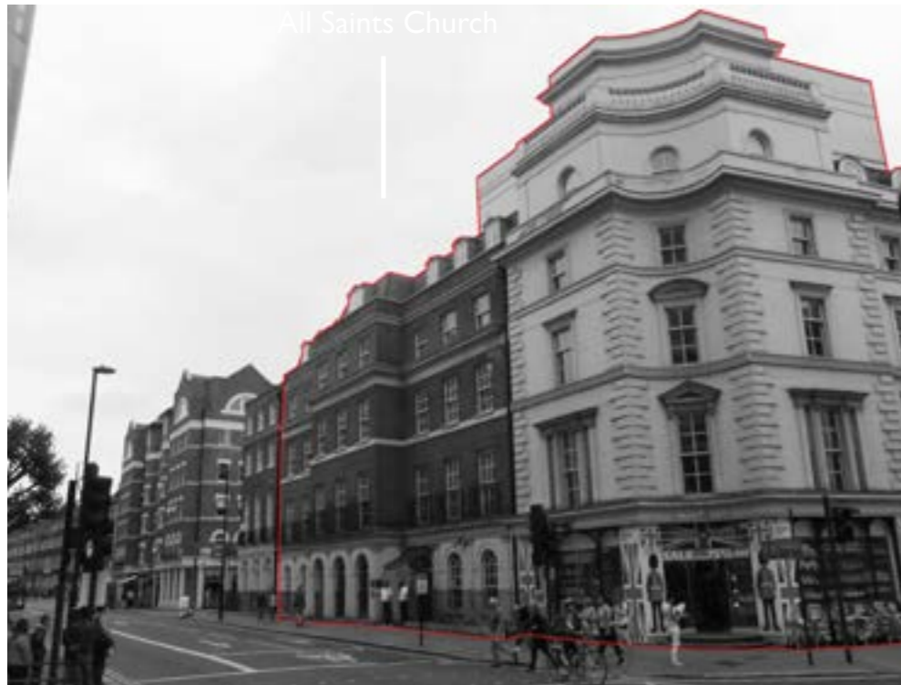
3. Looking North at the Junction of Bloomsbury and New Oxford St
