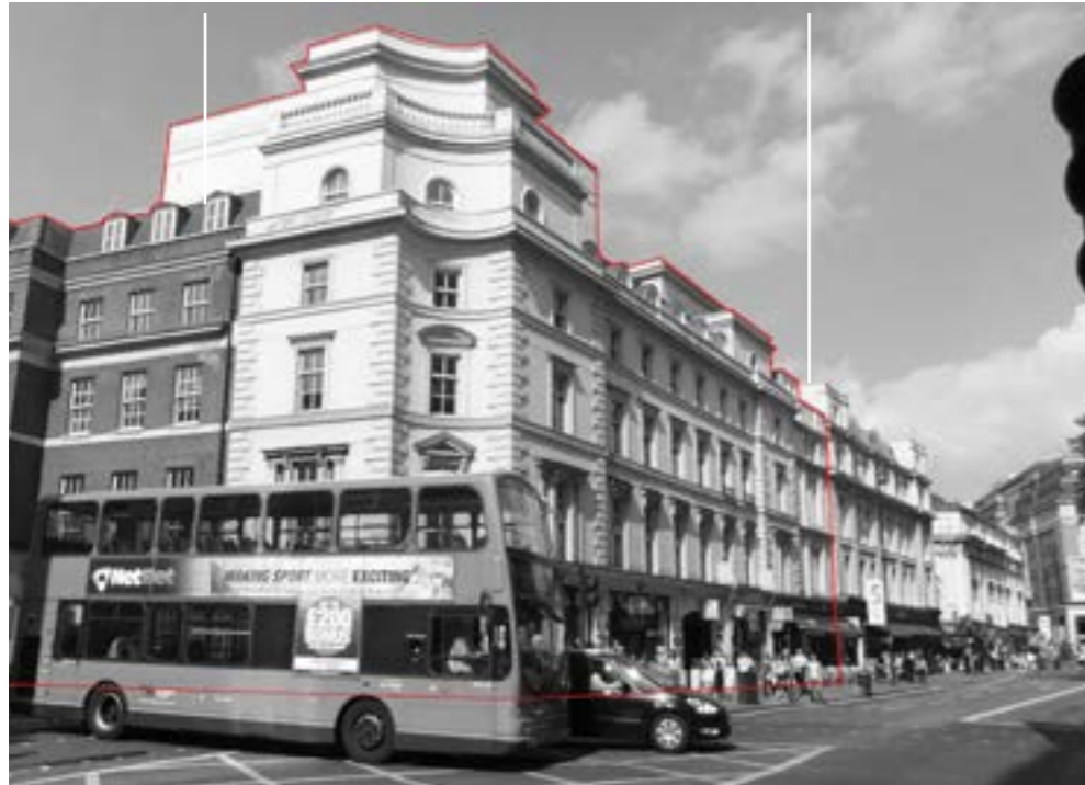
1. Looking East along New Oxford St Showing Inclined Curve Corner Treatment
