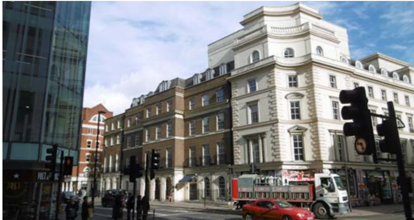
Existing Photo 1 - View looking North
