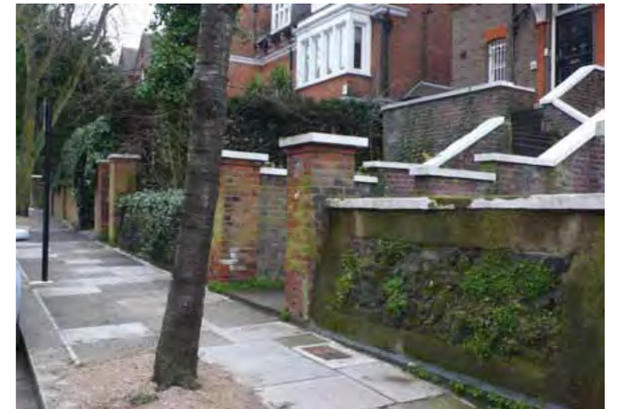
Fig. 2.3.2 North facing detail view of entrance steps
