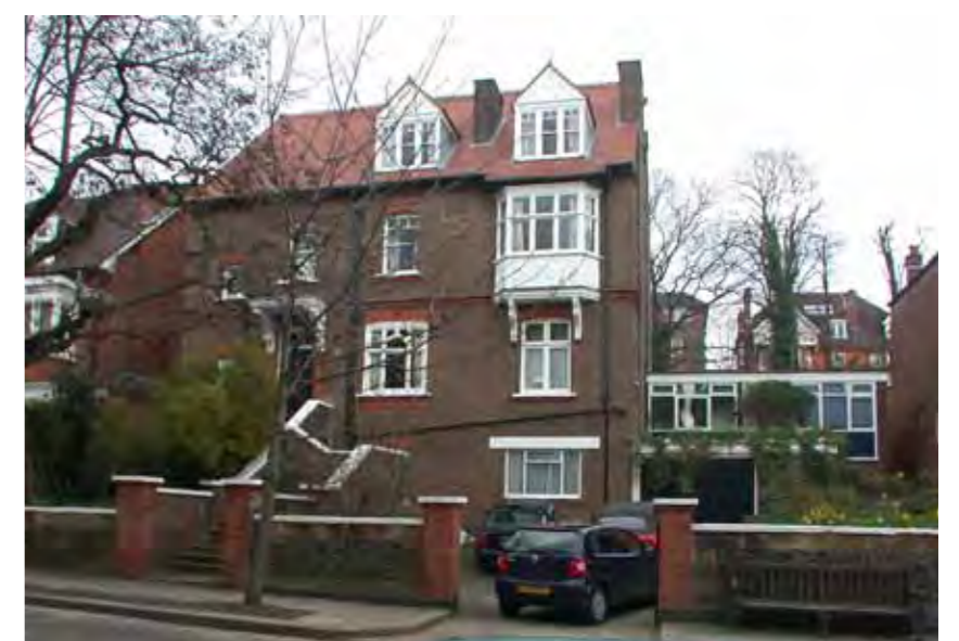
Fig. 2.3.4 View of the poor relationship between extension and original building
