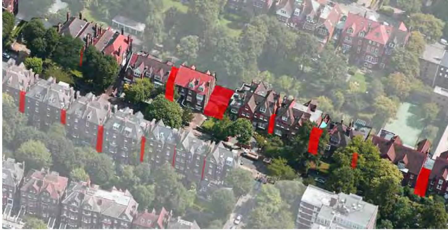
Fig. 4.2.9 Existing building widths, north-east view
