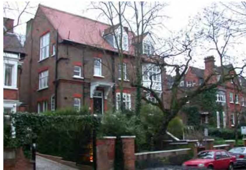
Fig. 2.3.1 South-east view of existing building
