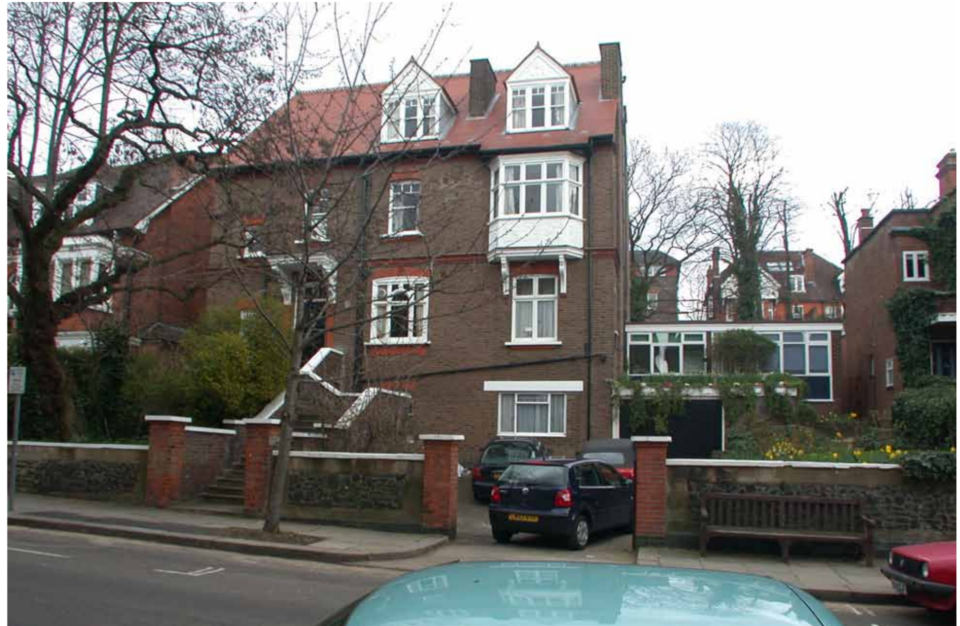
Fig 1.1.1 View of existing building at 26 Netherhall Gardens
