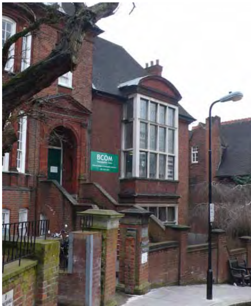
Fig. 4.3.7 No. 50 Netherhall Gardens, statutorily listed at Grade II
