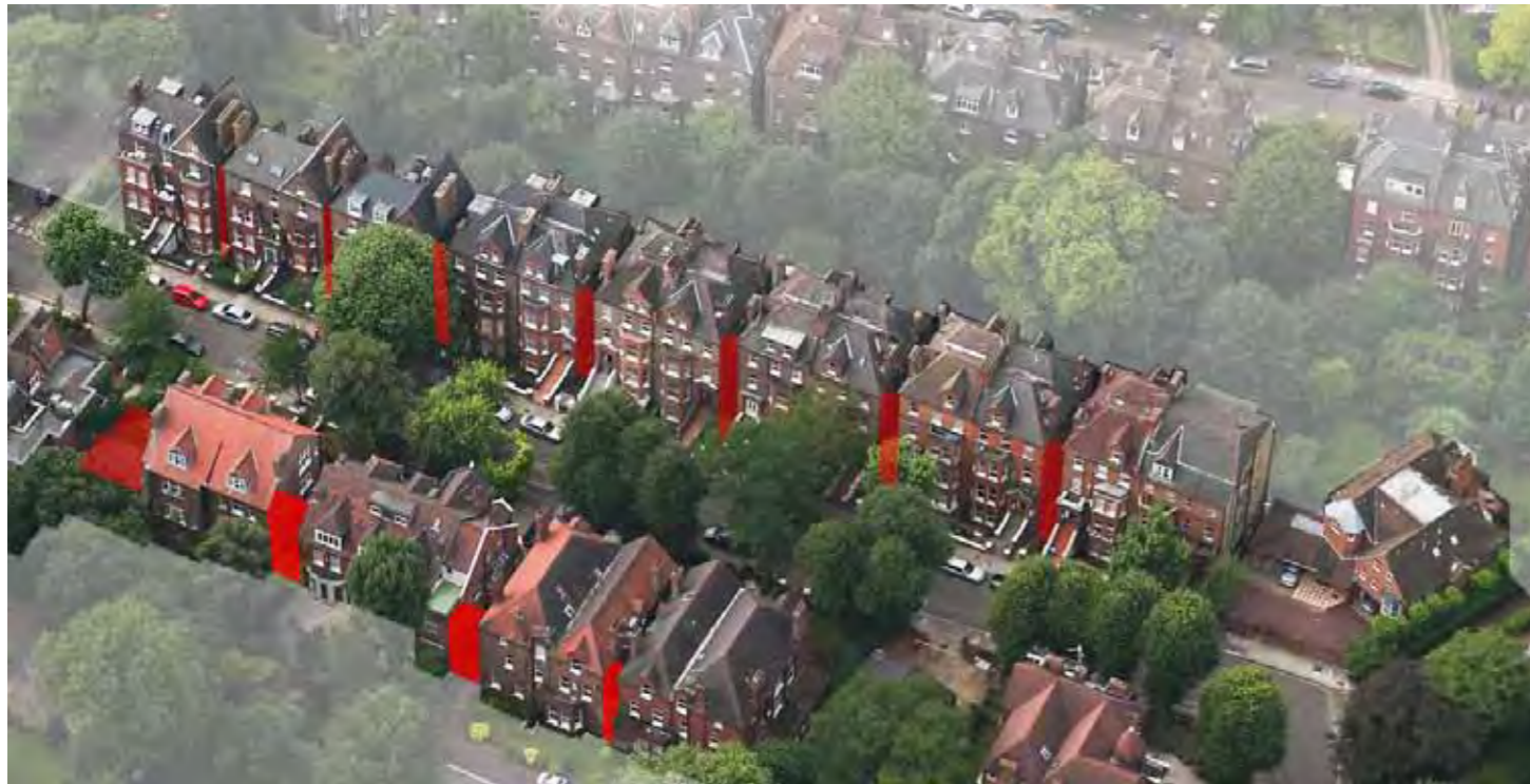
Fig. 4.2.10 Existing building widths, south-west view
