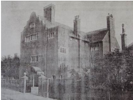
Severn House (demolished)
