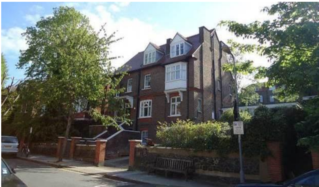
No. 26 Netherhall Gardens with visible southern flank and the 'gap' seen from the street
