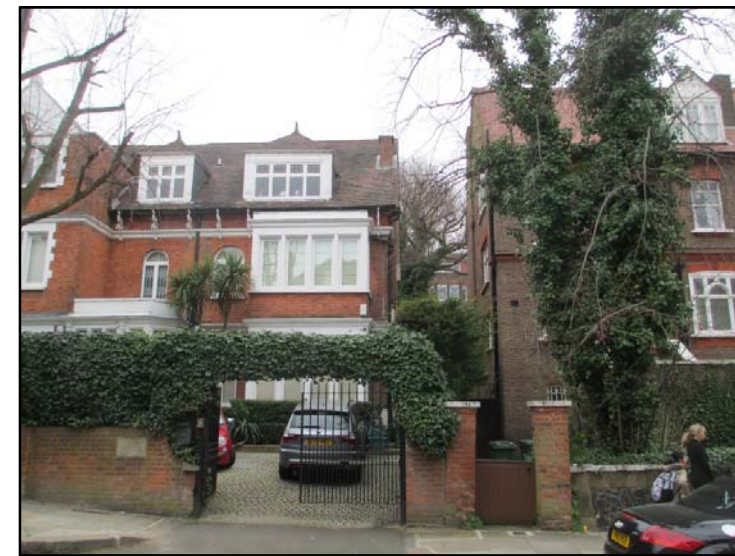
Photo 3: No 28 Netherhall Gardens
