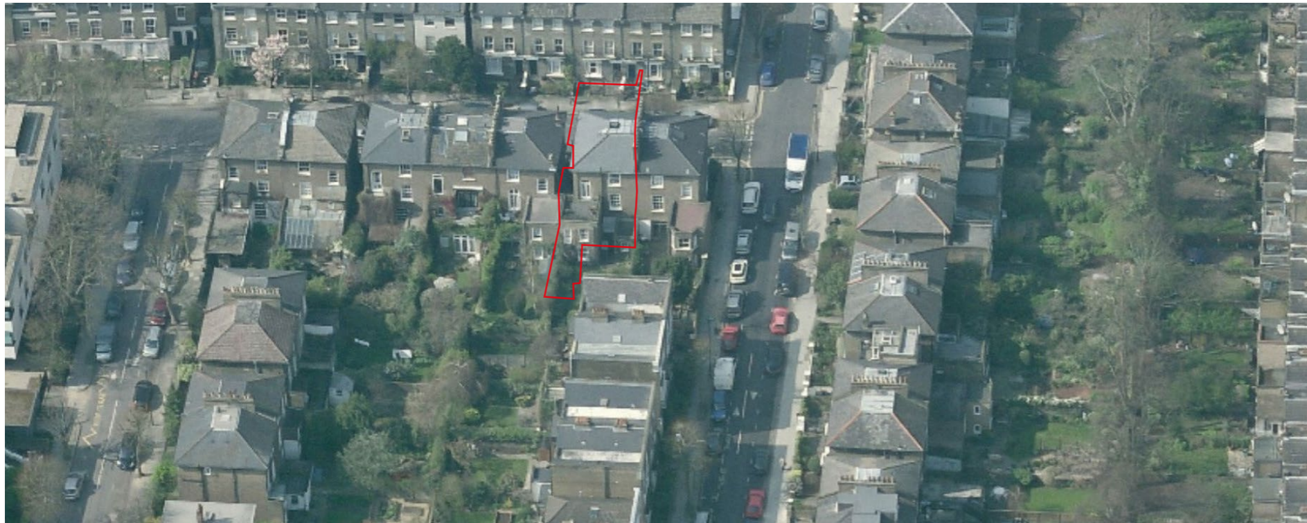
19 Bartholomew Villas outlined in red. No. 21 to the right. Existing one and two storey flat-roofed rear annexes.
