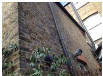
Flank of closet wing
