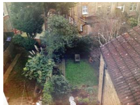
Boundary condition - towards rear
