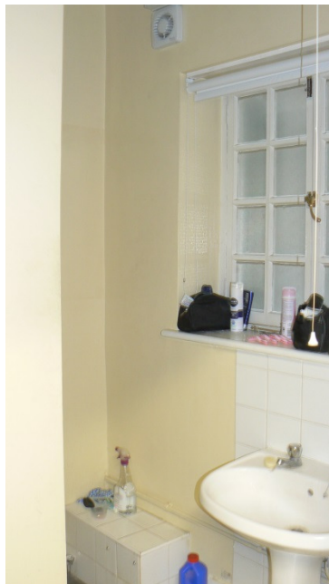
Existing shower room to be converted into a counselling room.
