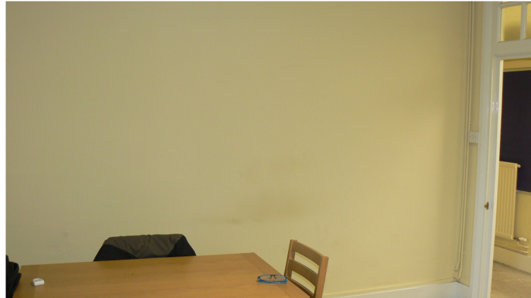
Lounge side of the wall where opening is to be formed.
