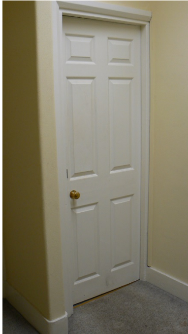
Toilet to be extended to accommodate wash hand basin.
