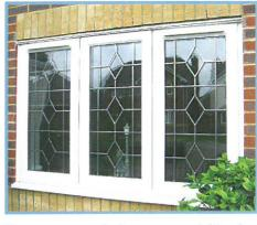
To create equal glass areas within the window design, it is necessary to introduce 'dummy sashes'.
