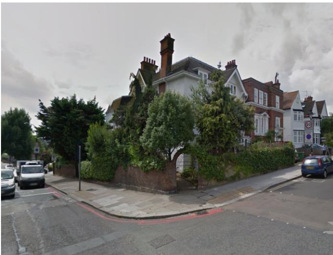
Photo G: View from Fortune Green Road & Ardwick Road
