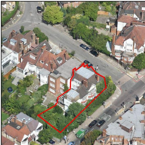
View facing north
