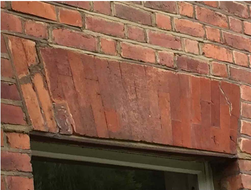
Cracking In Brickwork Arch Next Door
