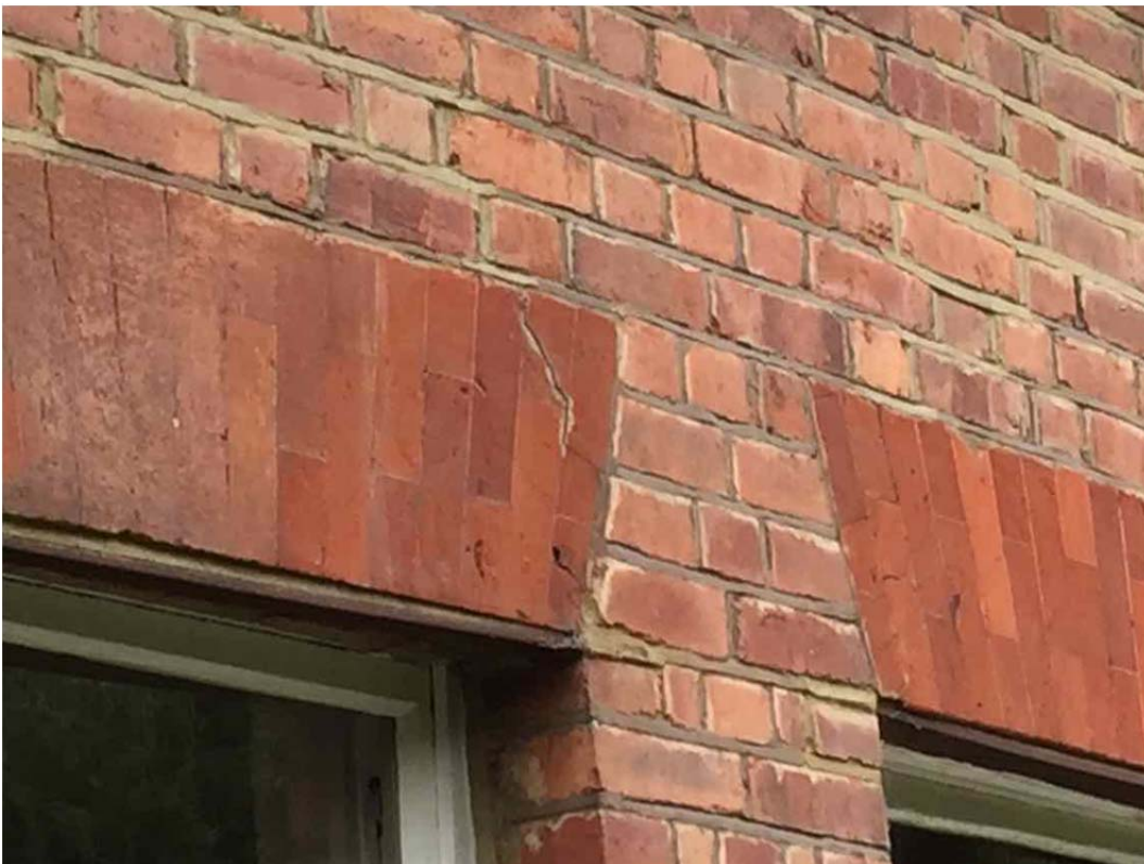
Cracking In Brickwork Arch Next Door
