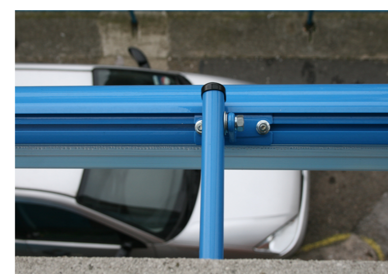
Below is a photo of the existing Microlux Slimline strip sign lighting from above. All light is directed downwards. Microlux Slimline strip sign lights by Portland Lighting Ltd. website: www.portlandlighting.co.uk
