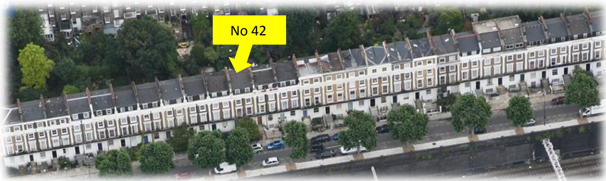
Fig 2: Mornington Terrace – listed row – Nos 26 - 52
