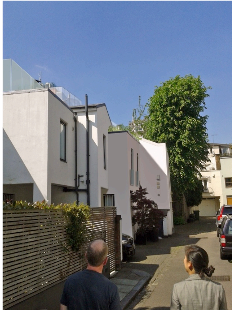
Fig.4 – Indicative montage showing how the proposed terrace will compliment the staggered aspect of the existing building.
