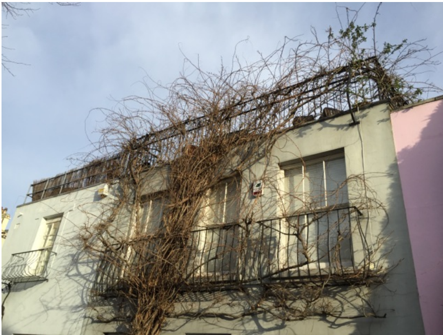
Fig.9 – Image showing the existing roof terrace at no.8 Albert Terrace Mews, opposite the application site.
