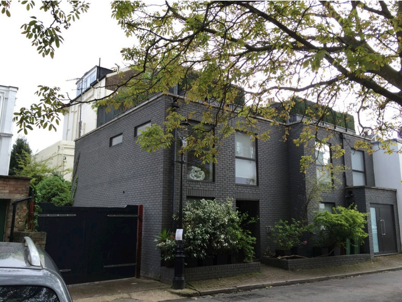
Fig 18 – Image showing the view of the roof terrace at No17 from the (East) Regents Park Road entrance to the mews.
