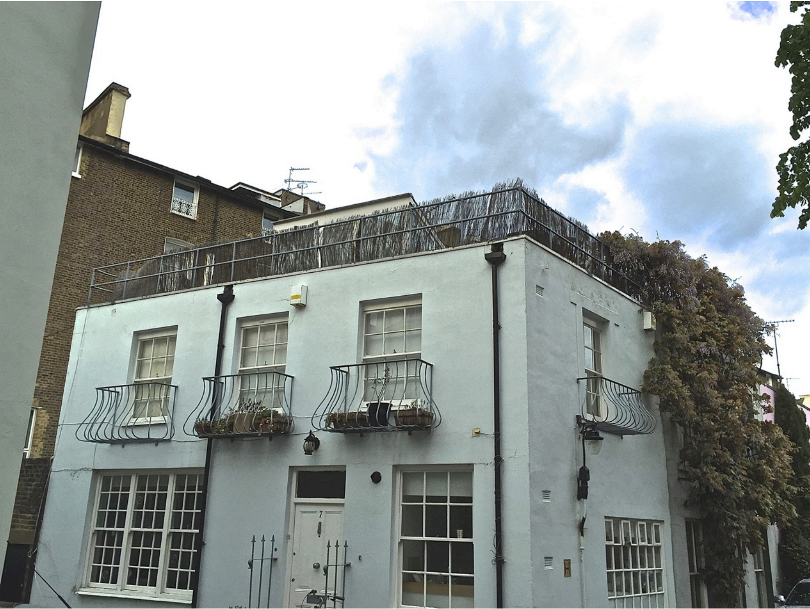
Fig 19 – Image showing the prominence of the roof terrace at No7
