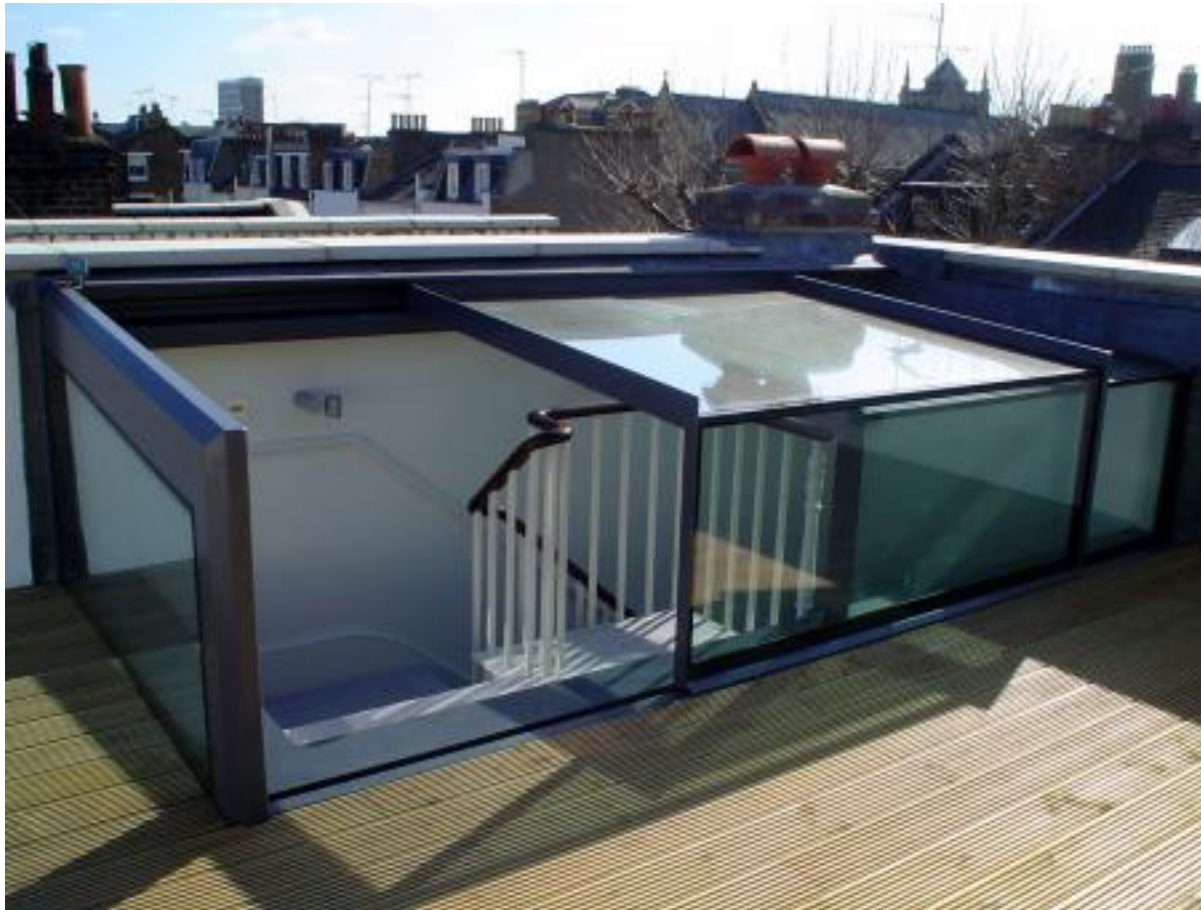
Fig.3 – Low lightweight structure for proposed roof access.
