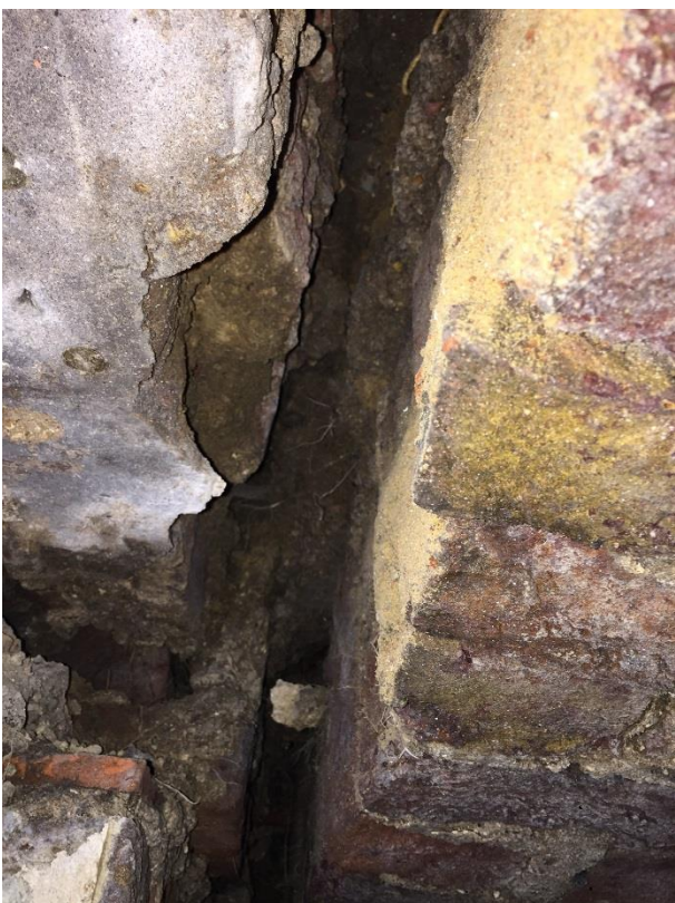
Photo No. 2: Gap between Existing vault and front wall.
