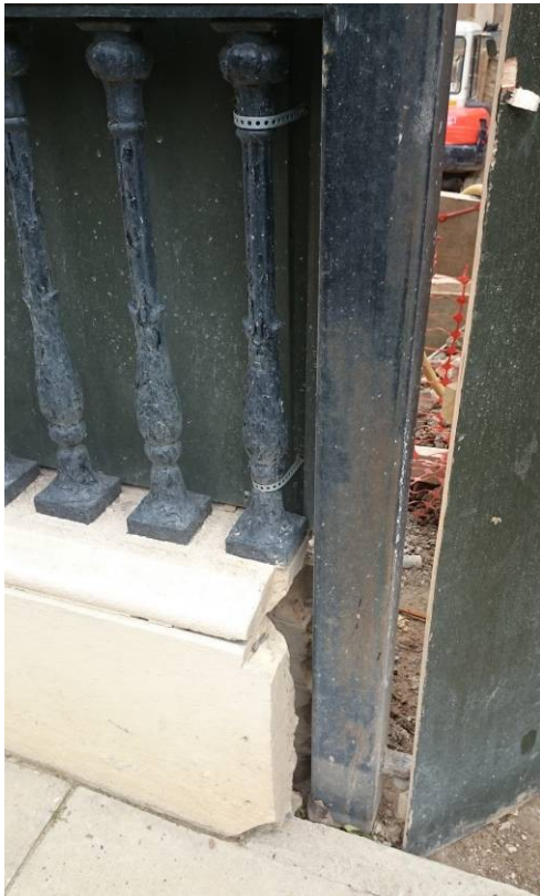
Fig 1. Cavity wall construction visible
