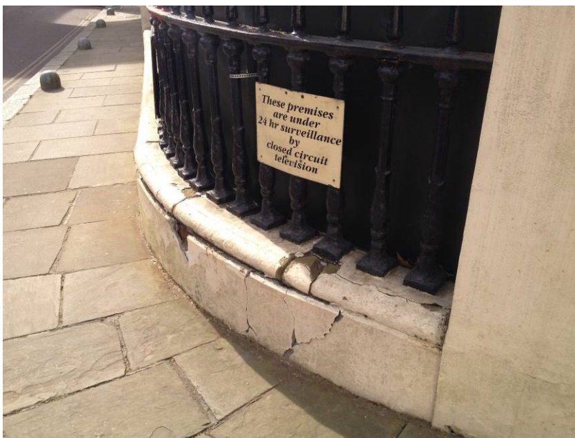
Fig 3. North boundary wall - first bay adjacent to the corner (N-W corner)
