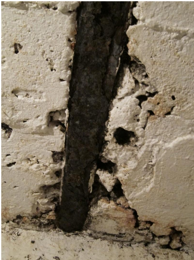
Heavy corrosion to steel
