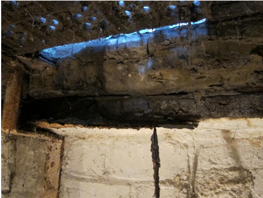
Steel trimmer virtually disintegrated
