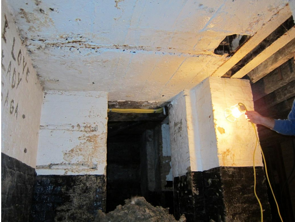
Typical view of vaults showing leaks, honeycombing to concrete and corrosion of steels
