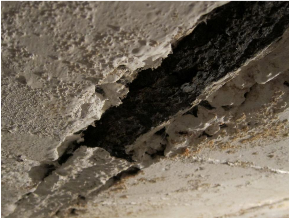
Delaminating flange of steel joist
