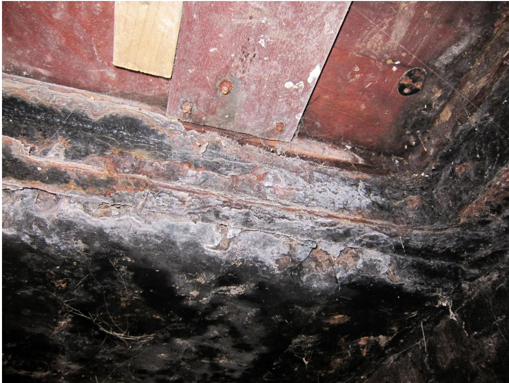
Heavy corrosion to steels around openings
