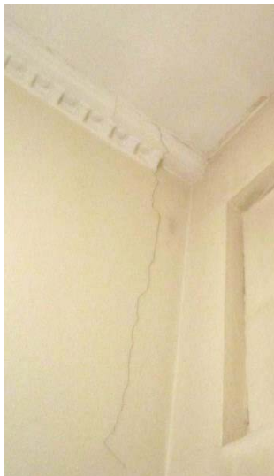
First floor – Crack in walls and ceiling to be repaired
