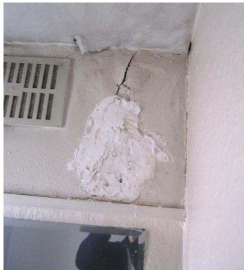
First floor – Crack in walls and ceiling to be repaired
