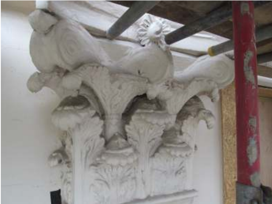
South Elevation Capital prior to application.
