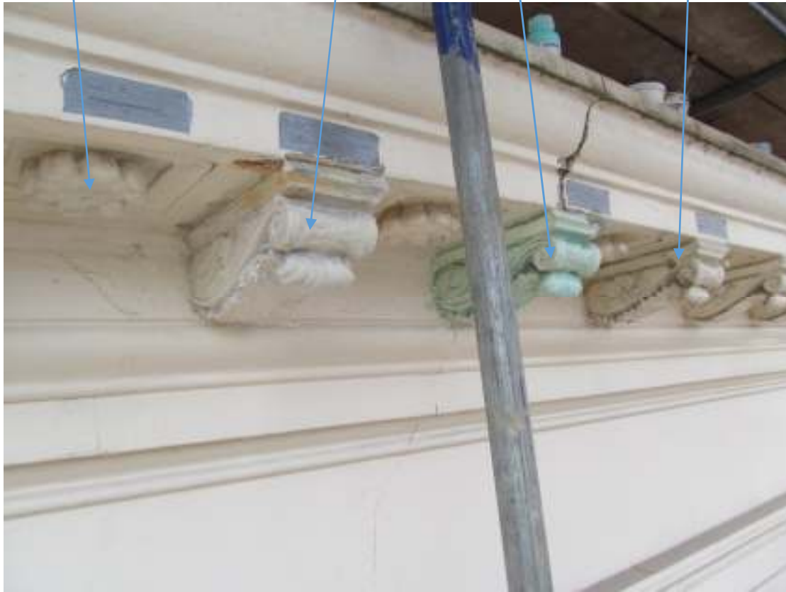
Application of chemical paint softeners
